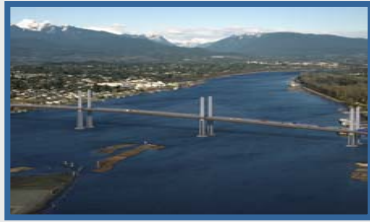
Golden Ears Bridge , Canada
